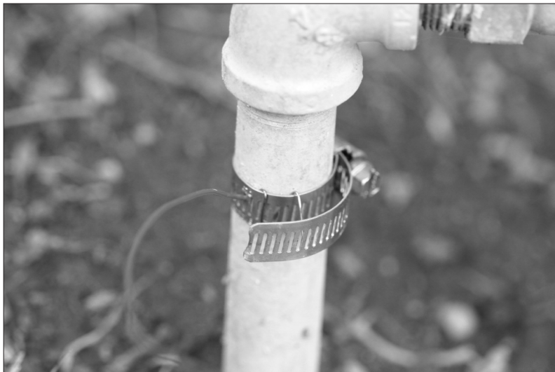
Figure 2-6: A good ground connection.
